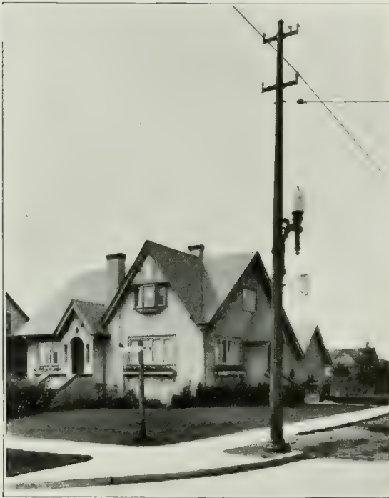
A Pole Designed to Carry Street Lighting Fixture and Power Wires, as Well as Acting as a Support for Street Railway Wiring.
